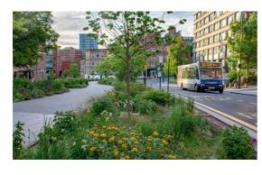
The Grey to Green scheme in Sheffield is the UK's largest retro-fit SuDS project, and also the UK's largest inner city 'Green Street'. One of the main functions of the Grey to Green scheme is to reduce and slow down surface-water runoff in an area of the city prone to flooding. Designed with climate change, wellbeing and economic investment in mind, Grey to Green is helping to lay the foundations for a healthy and sustainable urban future for Sheffield.
